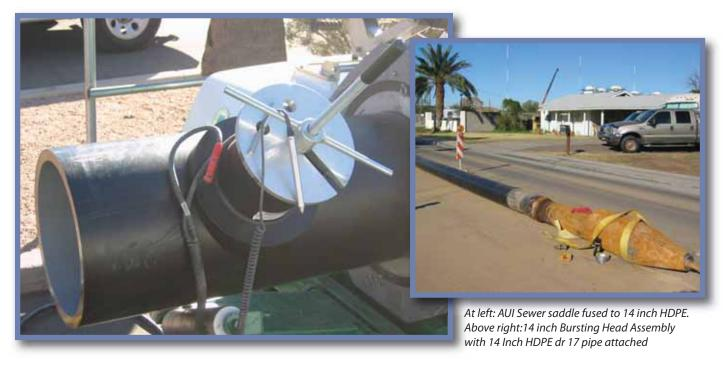
when passing through the existing sewer manholes) due to the substantial increase in pipe size, almost double the pipe size from 10 to 18 inches. The pipe bursting team completed all three pulls in 26.5 hours and completely replaced this segment of the sewer main in under ten days (including sewer lateral reconnections and surface restoration). This segment included a burst directly across an arterial, signaled intersection with no lane drops; completely undetectable to the traveling public.
