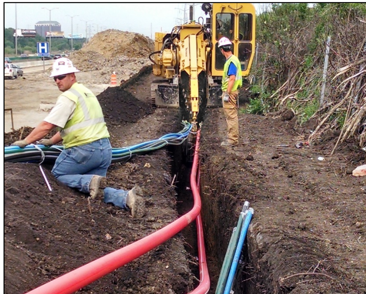
Figure 1: Open Cut Continuous Trenching Installation of HDPE Conduit
