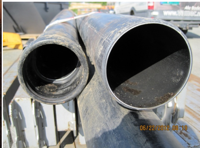
Figure 4.9.3 Excavated 110mm PP solid wall pipe from Vanvikan Norway, Pipe N1
