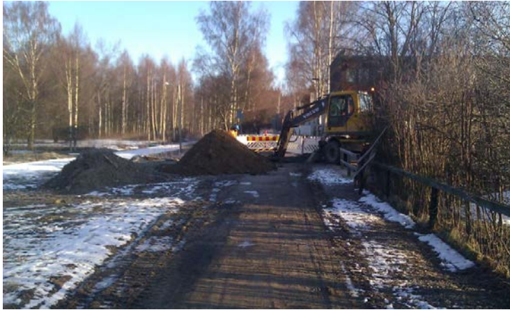
Figure 4.1 Location of the excavation site in Vaasa Finland, Pipe F1
