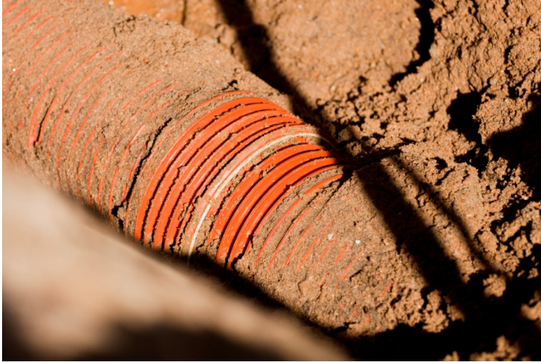
Structured-Wall pipe in the trench
