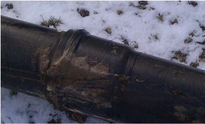
Figure 4.3 Excavated pipes, PE 200mm in Finland, Pipe F1
