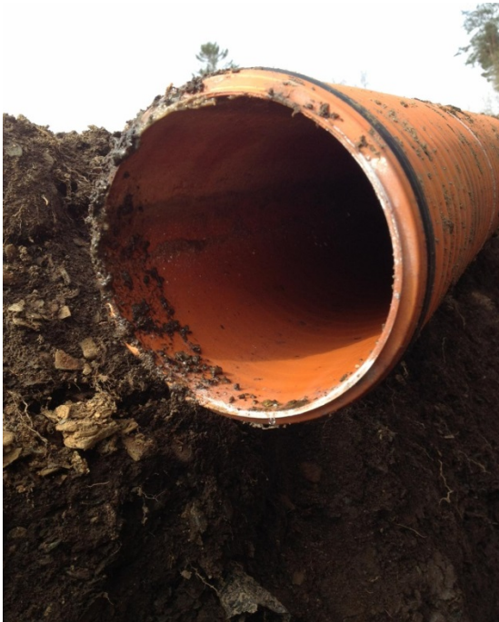
Excavation of 160mm structured-wall pipes in Surnadal Norway, Pipe N2
