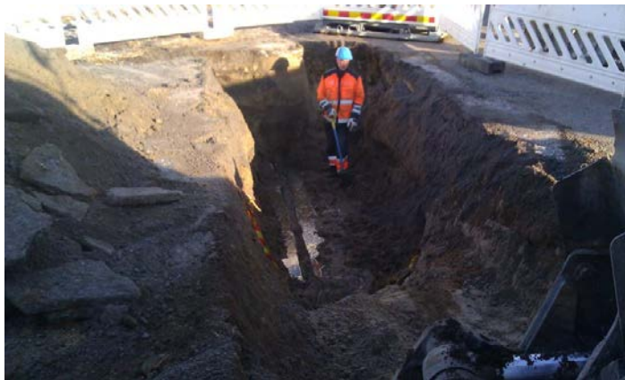
Figure 4.2 Excavation work, Pipe F1
