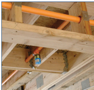
Home sprinkler heads during installation.
