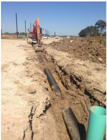
The pipe used at Youngsville also provided an environmental advantage. The MEGA GREEN® Series of Advanced Drainage Systems, Inc. (ADS) (Hilliard, Ohio) N-12® corrugated HDPE pipe is made with at least 40 percent recycled content. More than 23,800 linear feet of the pipe in diameters ranging from 10 to - 48 inches was used on the project. MEGA GREEN pipe provides both strength and optimum hydraulic capacity with a Manning's "n" rating of 0.012. It meets ASTM
