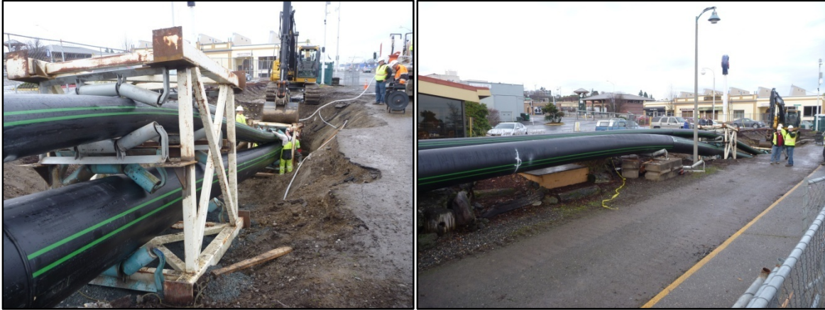
Figure 6. Insertion of 30-inch and two 14-inch pipes using bundling/taming frame.
