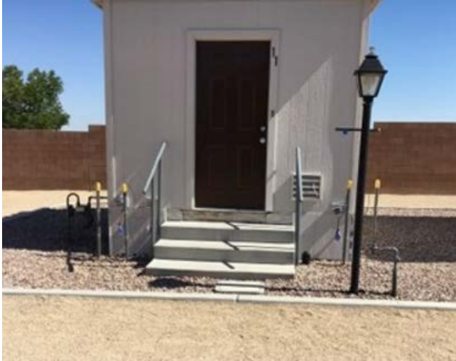
Figure A.5: Henderson, NV service risers (south facing)
