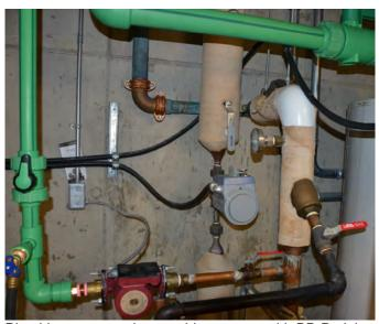
Plumbing systems that combine copper with PP-R piping materials are appropriate as long as the flow rate within the copper components is not excessive, according to the Plastics Pipe Institute.
