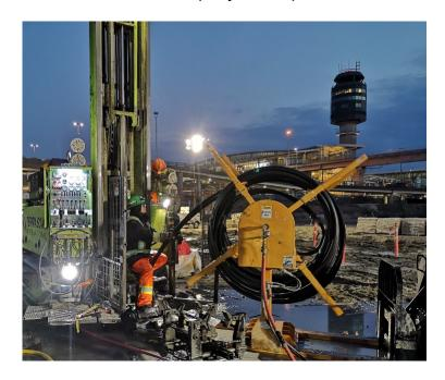
The Vancouver International Airport's new Central Utilities Building (CUB) will improve efficiency by centralizing all of the equipment needed to meet the airport's heating, cooling and electrical demand. To achieve this goal, the project will rely on one of the largest Geoexchange systems in Canada. Geoexchange technology uses the earth's renewable energy, just below the surface, to heat or cool buildings. This system will provide sustainable heating and cooling for the terminal.
