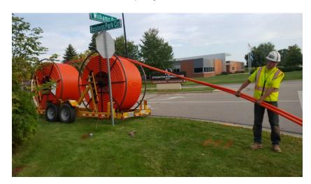
Teel conduit is being installed across Alliant's service area in lowa and Wisconsin to improve its telecom network's security, speed, and reliability. For a utility with a large service area including more than 970,000 electric and 420,000 natural gas customers, reliability and capacity are is crucial during critical events. The conduit will protect the existing infrastructure and allow for later expansion of network capabilities while providing cost savings to Alliant Energy.
