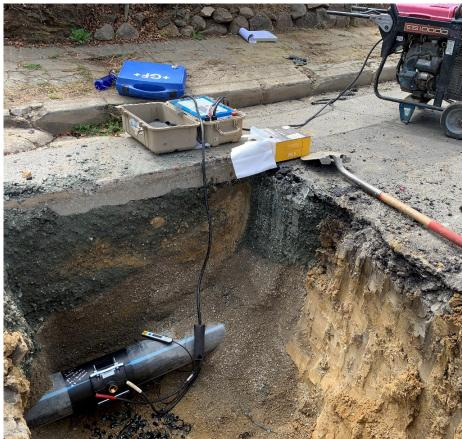
The procedure for repairing a tapping saddle on an HDPE pipeline, as well as other methods, is detailed in the free document, *MAB Basic HDPE Repair Options – MAB-4,* from the Municipal Advisory Board.
