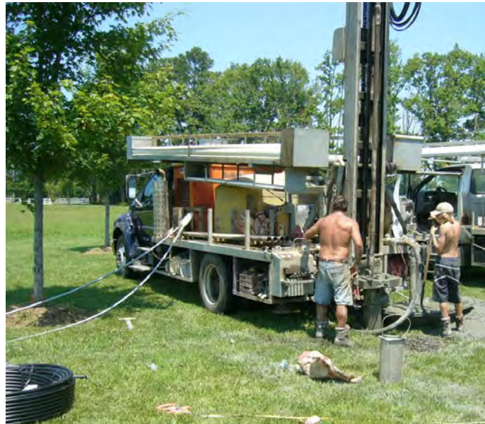
A geothermal system being installed.
