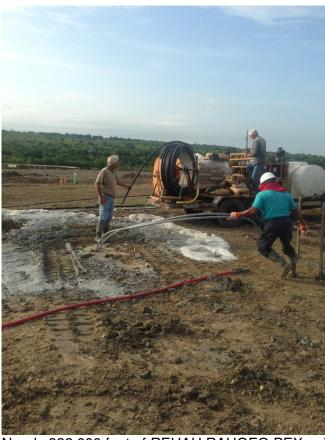
Nearly 322,000 feet of REHAU RAUGEO PEXa pipe was used to produce the 237 double U-bends, which were inserted into each borehole. The crosslinked polyethylene (PEXa) pipe is specifically designed for geothermal applications.
