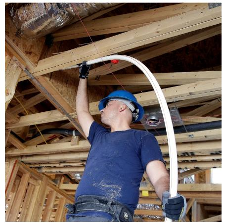
Available free on PPI's website, TN-56 *Installation of Plastic Pressure Piping Materials Near IC-Rated and Non-IC-Rated Recessed Lighting Fixtures* provides guidance to installers of plastic piping materials about protecting these piping systems against excessive heat through sufficient distance, insulation, or other means.
