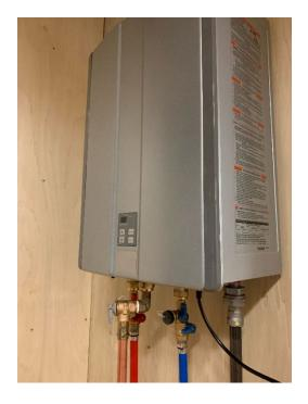
Available free on PPI's website, Recommendation H "Direct Connection of Plastic Piping Materials to Tankless Water Heaters for Domestic (i.e. residential) Applications" provides guidance about direct connection of piping materials CPVC, PEX, PE-RT and PP to tankless water heaters.
