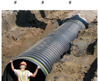
Some corrugated high-density polyethylene (HDPE) pipe is made with a minimum of 40 percent recycled content, taking bottles from curbside collection to lifelong underground infrastructure improvement.
