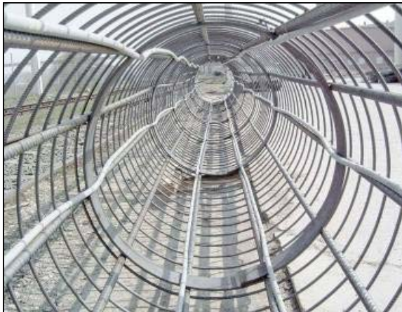
PEX in rebar cage/structural pile
