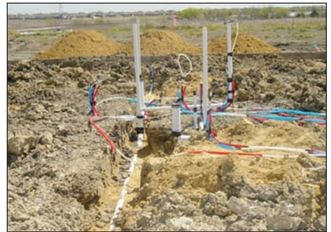
PEX pipe beats copper in areas where aggressive water causes pinhole leaks and system failure.
