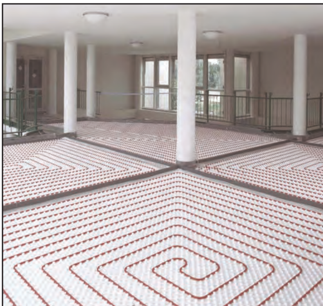
Figure 11.1 – Radiant Floor Heating Piping in a Residential Application
