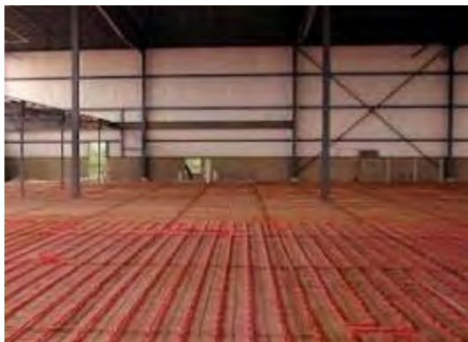
BCD: PEX tubing for radiant heating
