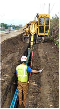
HDPE conduit is popular for installing underground cables on DOT projects. PPI's MS-5 Model Specification references appropriate standards for specifying HDPE conduit for power and communications projects.
