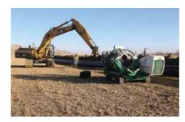
was installed using traditional open cut trenching with a few horizontal directional drills at river crossings.
