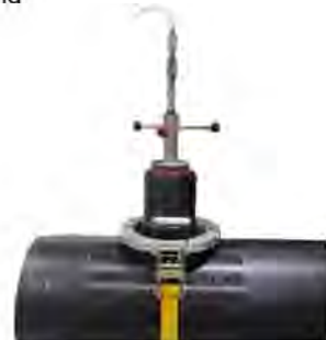
7. After observance of cooling time and prior to tapping main, saddle should be pressure leak tested. It is recommended to use hydrostatic testing whenever possible. Care must be exercised during pressure testing of saddles due to the stored energy of the test fluid. Pipe plugs or other sealing mechanisms should be restrained to avoid expulsion and possible safety related issues associated with this procedure. Refer to ASTM F2786 when performing pneumatic tests.
