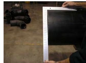
Figure IV-b - Measuring allowable gap with Carpenter's Square
