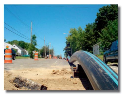
City engineers estimated that using HDPE pipe meant the project was completed in about 60 percent of the time it would have taken with traditional excavating. Moreover, the resulting re-paving was completed with just two inches of asphalt instead of 10 inches of concrete and four inches of asphalt, due to almost no ground disruption.
