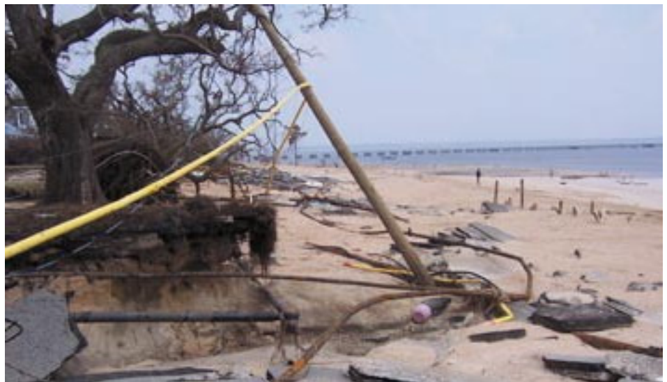
Gas lines strung up along the beach in Bay St. Louis, Mississippi.
