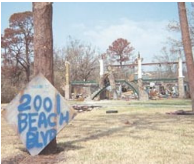
This was built on pilings to deal with flooding. It didn't work.
