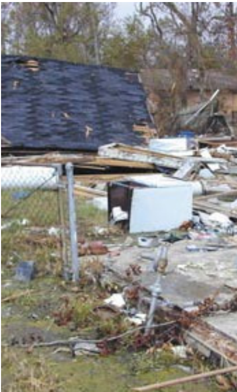
All that is left of this house in Pascagoula is a concrete slab, a metal fence, and the gas riser.
