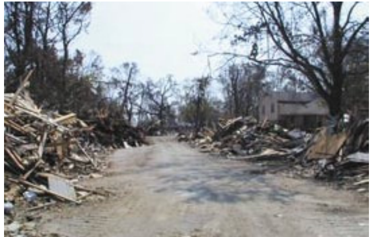
Mountains of debris pushed aside to clear a path through the streets.
