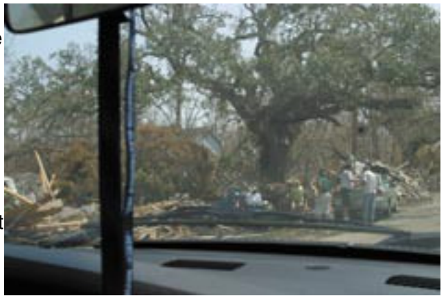
Residents are seen returning to the devastated 1/2 mile of coastal Waveland to salvage whatever they can from the wreckage of their houses. This is the view from one of the gas trucks on during an early visit to the area.
