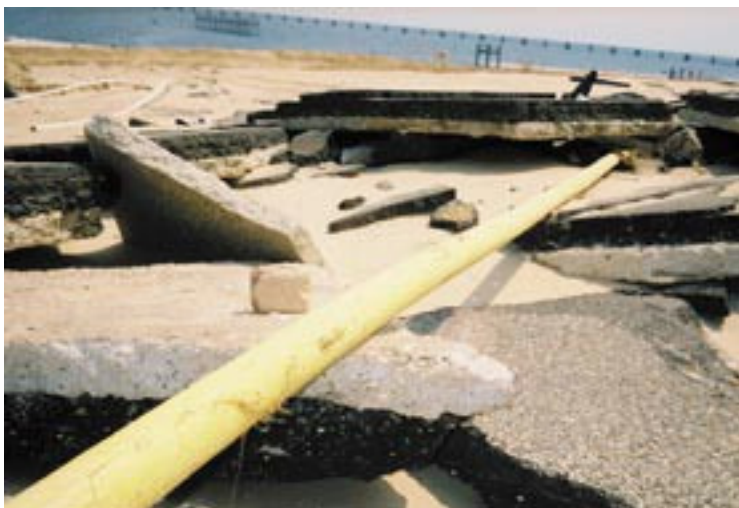
Asphalt and natural gas pipe bear mute witness to the power of Katrina in Bay St. Louis. In the background are the pilings of the railroad bridge across St. Louis Bay.
