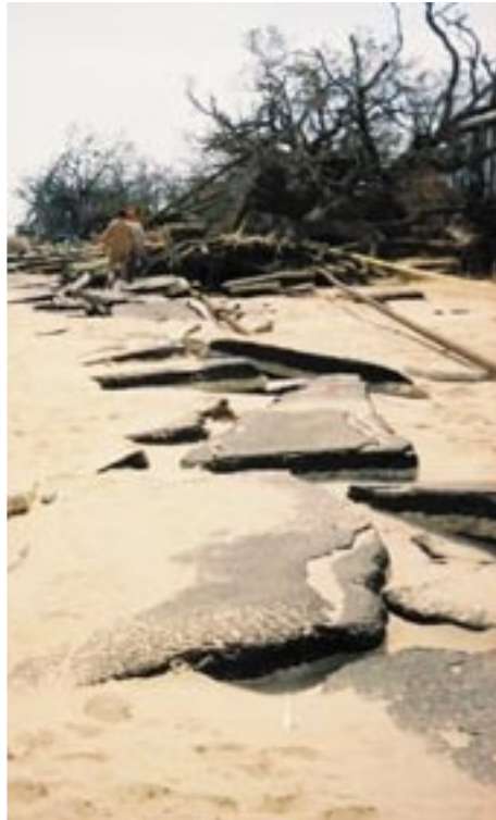
This was once a city street, with a gas main under the shoulder.
