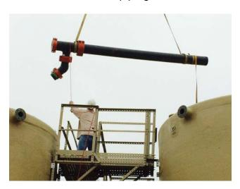
The original plan called for the pipe to be fused, but the fusion process presented several challenges for this project. The tight spacing between the tanks combined with the larger diameter piping would have required some of the fusing to take place away from the tank battery, and for the spools to be hoisted in and mechanically joined. There was also a risk of the fusion equipment damaging the liner in the containment area. To overcome these difficulties, Atlas Resources decided to use
