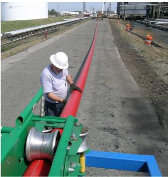
Available for free on PPI's website, TN-61 "*Coilable HDPE Conduit Ovality and Coil-set*" provides information about what can cause ovality and coil-set in HDPE conduit products, and describes measures that can be taken to correct or reduce ovality during installation.
