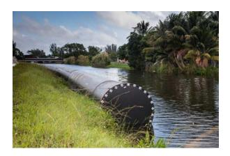
On the ends of the line, connections were made by flange-to-valve. There were also 48 air release valves (ARVs) and access manways that needed to be installed on the 63-inch line within the host pipe. ISCO supplied the HDPE PE 4710 pipe manufactured by JM Eagle (Los Angeles) and worked with Ric-Man to make the ARVs and the manway connections to the HDPE.
