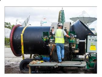
Design pressure for the pipeline was 65 psi with operating pressure of 10 - 25 psi. The 20-foot sections of the five foot diameter HDPE pipe were heat fused together using a McElroy MegaMc® 2065 unit. Cover depth for the pipe ranged from three to four feet. JM Eagle and McElroy are also member companies of PPI.
