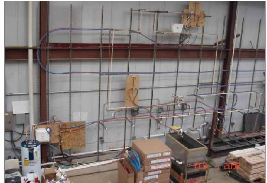
Figure 8.2 – Laboratory Test Set-up with Five Outlets, Hot Water Tank, and T&B System
