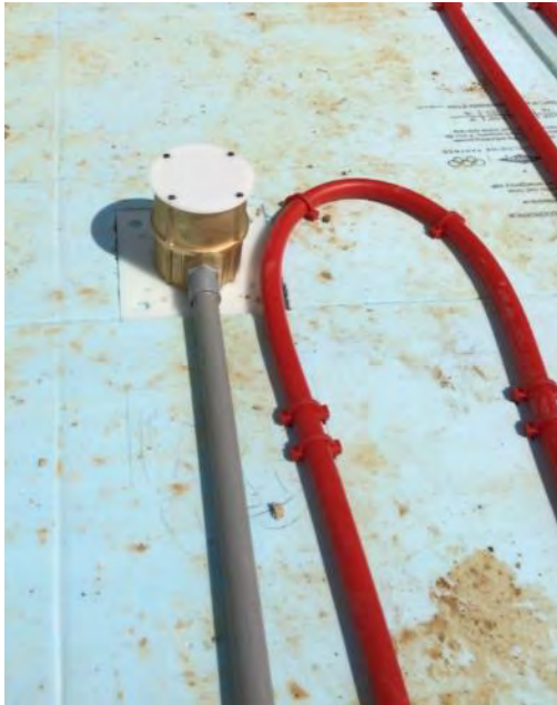
Sensor socket before concrete
