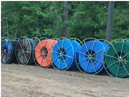
PCD: HDPE Conduit for fiber optic
