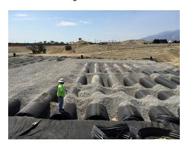
HDPE was selected over other pipe material alternatives for this job according to Currence. "We were told that the engineer typically considers both corrugated metal pipe and corrugated HDPE pipe for these types of projects, but prefers to use HDPE when there is no significant difference in price. He feels that HDPE pipe offers greater longevity."
