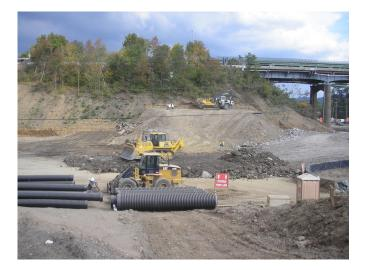
"Because each corrugated HDPE pipe section is around 20 feet long, there are fewer joints," Radoszewski explained. "This reduces labor and easily provides a secure system. Reinforced concrete pipe (RCP) comes in smaller 8-foot sections that weigh considerably more and so it would cost more to use and install than corrugated HDPE pipe."
