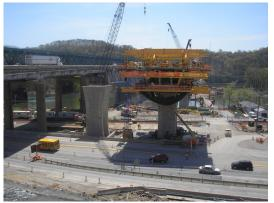
Twin bridges that are each 2,350 feet long, 61 feet wide and up to 120 feet high will be constructed as cast-in-place concrete segmental box girders. The new bridges will be downstream from the present span. The
