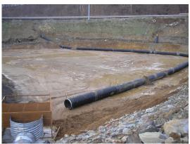
"The major part of the temporary diversion is on the north side of the project. We constructed a mountain of fill that's about 120 feet high. This eliminated a lot of existing drainage, and disturbed the water flow in that area. Water has to be diverted because we don't want water getting into the fill."
