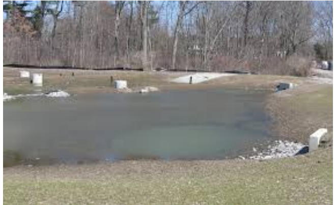
The gravel wetland detention basin at NHDOT I-93 Exit 2 Park-and-Ride is just one of the BMP techniques used to treat storm water runoff all along I-93.
