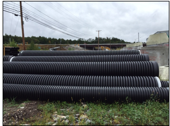
Corrugated HDPE pipe was selected for the storm water management system along I-93 due to its long life, ease of installation and cost effectiveness.
