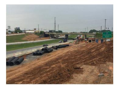
Currence elaborated on the properties of the pipe, "The HDPE material will not corrode, rust or degrade due to biological attack so the pipe resists bio-clogging and will be able to maintain high and consistent flow capacities over the service life of a system. And HDPE pipe has a very favorable strength-to-weight ratio.
