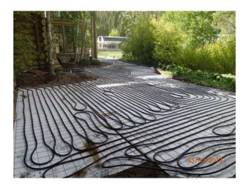
choice for radiant heating systems and is quickly replacing copper for residential potable water plumbing. In addition to outdoor snow and ice melt systems, other applications include AWWA municipal water service; turf conditioning; residential fire sprinklers; and geothermal systems. Typically found in sizes from 3/8 to 2 inches, and up to 3 inches in diameter, PEX pipe comes in straight lengths or coils and is made from proven high-performance materials."
