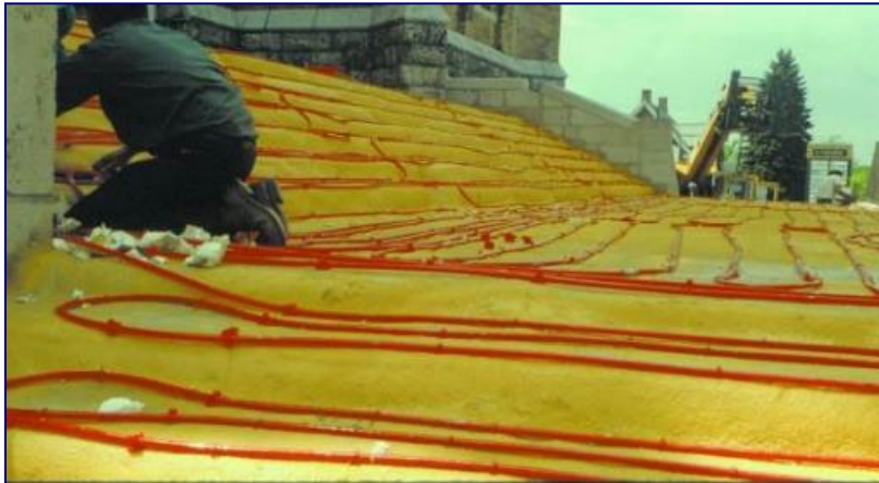
Spray-foam insulation on old stone steps (church)
