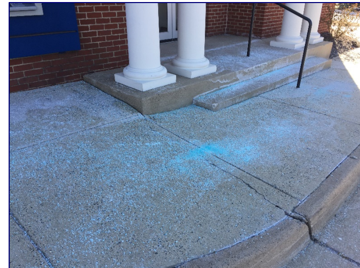
Salt at bank entrance
