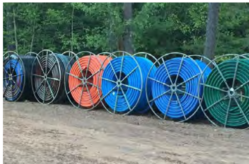
PCD: HDPE Conduit for fiber optic
