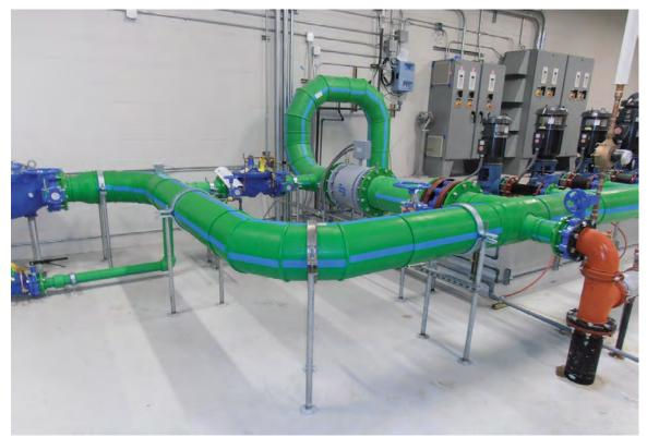
Polypropylene pressure piping in a commercial plumbing application. PPI's new Polypropylene Pressure Pipe Steering Committee within its Building and Construction Division (BCD) will focus entirely on polypropylene pressure pipe.
