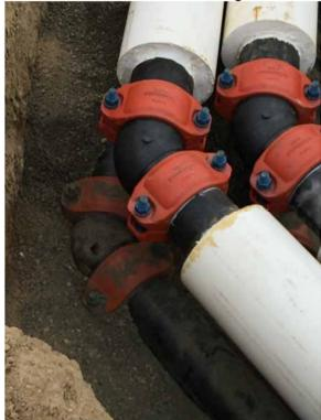
Without Victaulic's coupling technology, more than 75 percent additional labor would have been needed for the installation of the HDPE piping systems.
