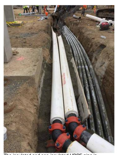
The insulated and non-insulated HDPE pipe is joined to *Victaulic* HDPE fittings using *Victaulic* Style 905 Couplings. A fully restrained system, *Victaulic* fittings and couplings are designed to be buried.
