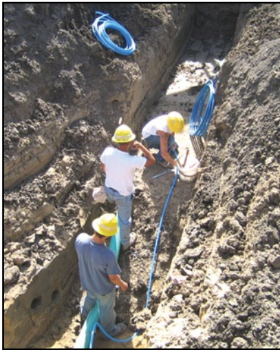
Figure 11.3 – PEX Water Service
