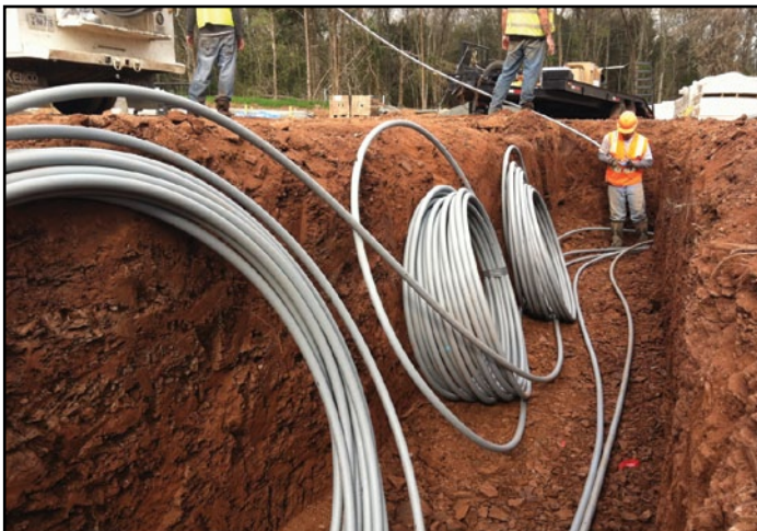
Figure 11.7 – PEX Piping in a Geothermal Application
